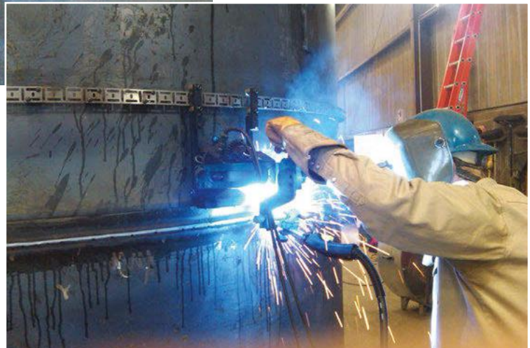
Li'l Runner with flex rail for tank fabrication.
